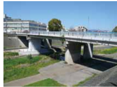
橋梁の耐震補強
